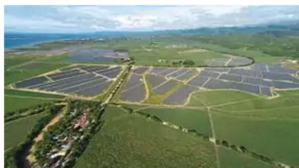
SaCaSol I solar power plant sa San Carlos City, Negros Occidental
