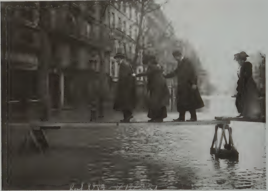
Figure 22. The Parisian Flood of late January 1910. Avenue Ledru-Rollin, January 30, 1910. Bnf.
