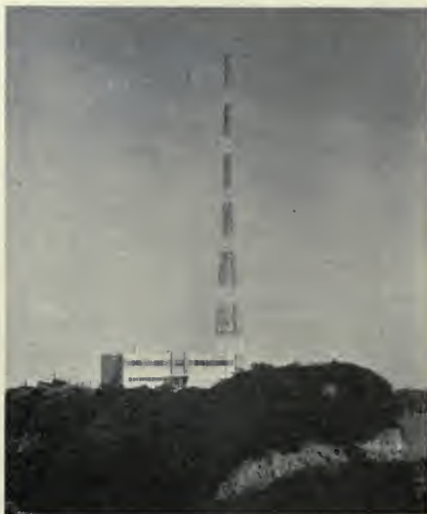
FIG. 1. The Mt. Lee television installation of the Don Lee Broadcasting System, Hollywood. This is the receiving location for all portable pick-ups where the incoming image on 324 megacycles is rebroadcast by station W6XAO . The tower is 2000 feet above sea level and the building houses all television operations.
